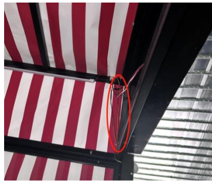
7.Link overhead white light bar to plug-in cable
